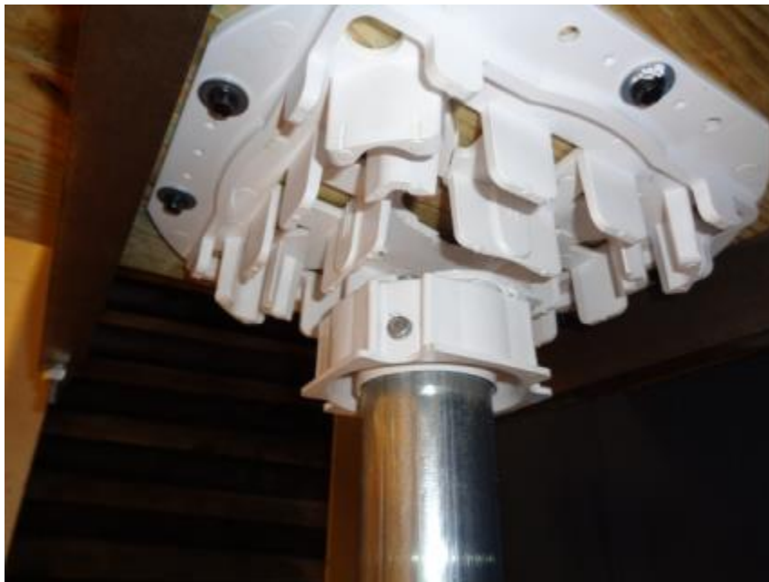
Photo No. 4 Typical Uplift Load Test Failure - 2-3/8 in Diameter Post
